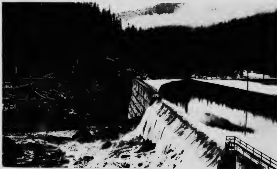
Vancouver Island Power Company Limited. Jordan River Dam with water passing over spillway.
